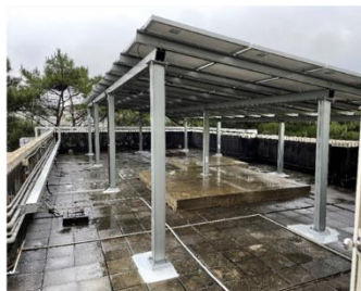
Installation of Solar Panel
